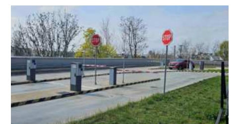
Šantovka Shopping Gallery, Czechia Parking in the shopping gallery - 2000 parking spaces, 3 parking areas within the building, 3 outdoor parking lots
